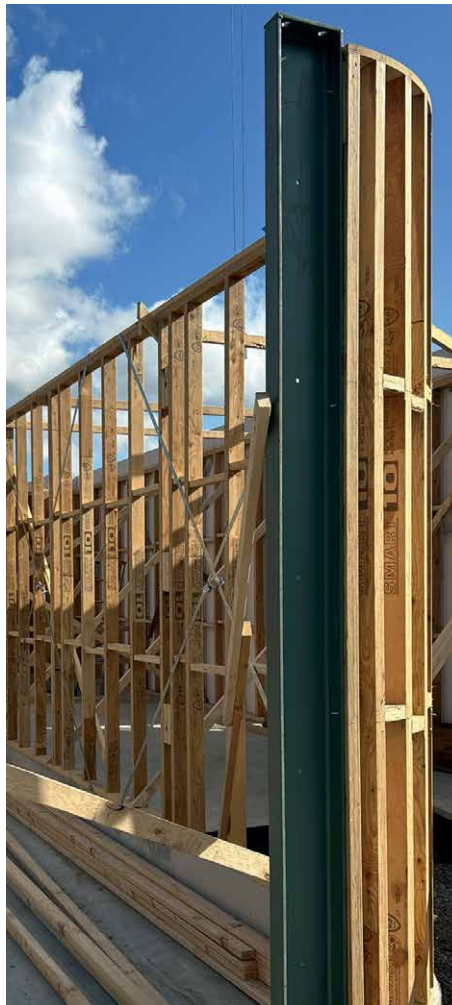
Above: Correctly detailed tall LVL wall studs including curve.
