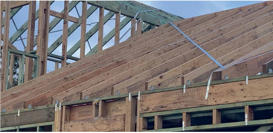
Above: Extensive use of LVL as studs, lintels and rafters.
