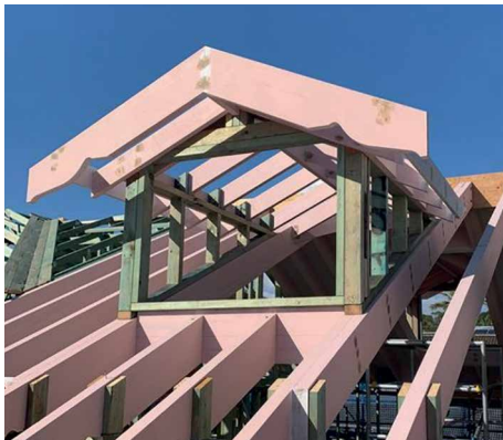
Above: Roof trusses constructed from Weatherproof.
