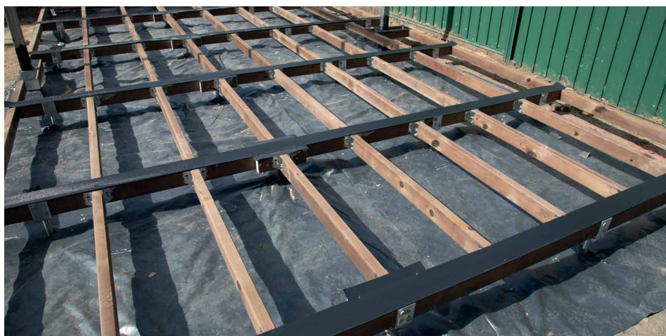
Above: Being timber, TerraFrame is easy for installers to use on site. Adding joist tape can help to move water away from the top of the subframe.
