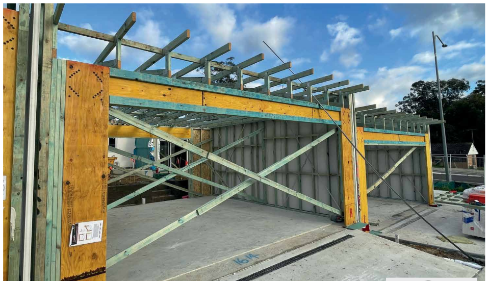
Above: meyBRACE, party walls, floor and roof cassettes all in one job supplier by the fabricator.
