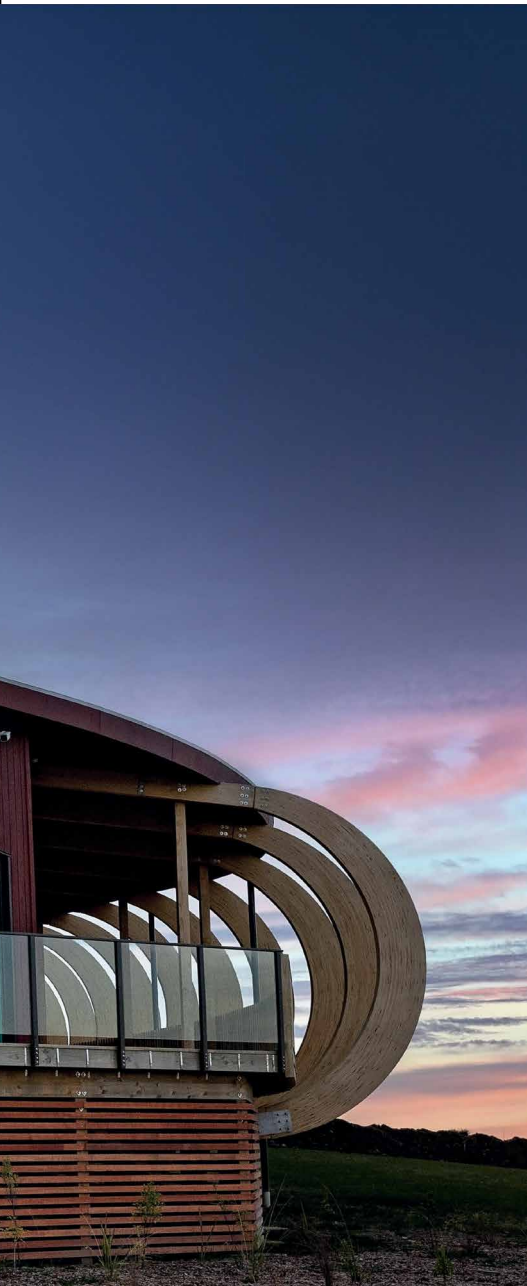
Above: Curved glulam beams make up the whalebone structural effect along one side of the building. Left: Murihiku Marae stands as a testament to sustainable building practices.
