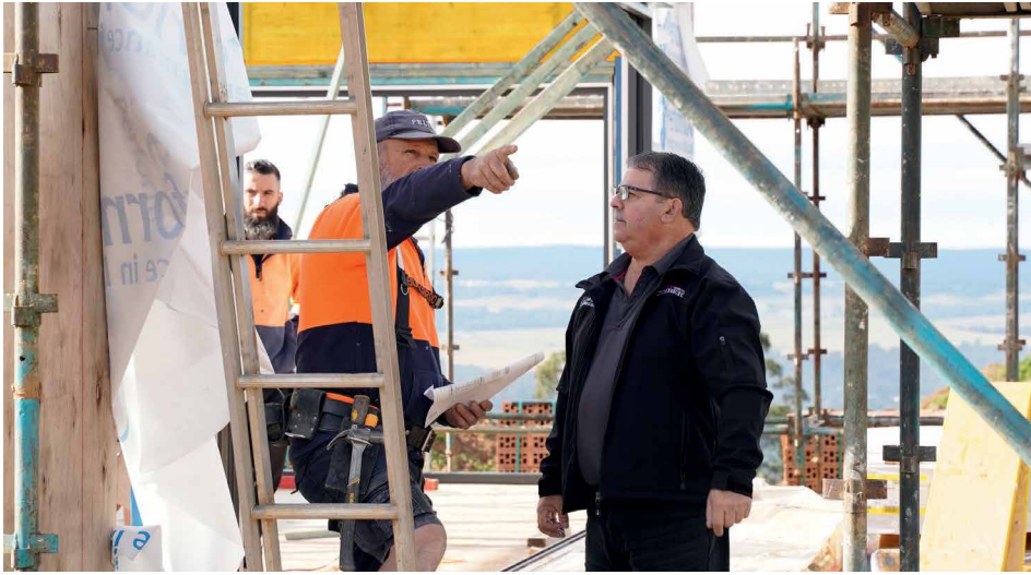
Above: Meyer Timber's 'Builder-go-to' Charlie Vella providing onsite support.
