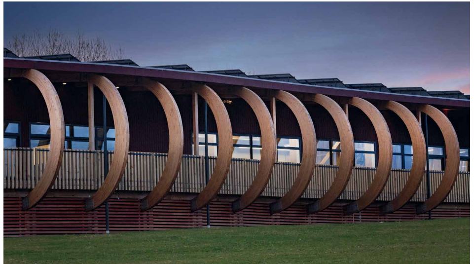
Above: Curved glulam beams make up the whalebone structural effect along one side of the building. Left: Murihiku Marae stands as a testament to sustainable building practices.
