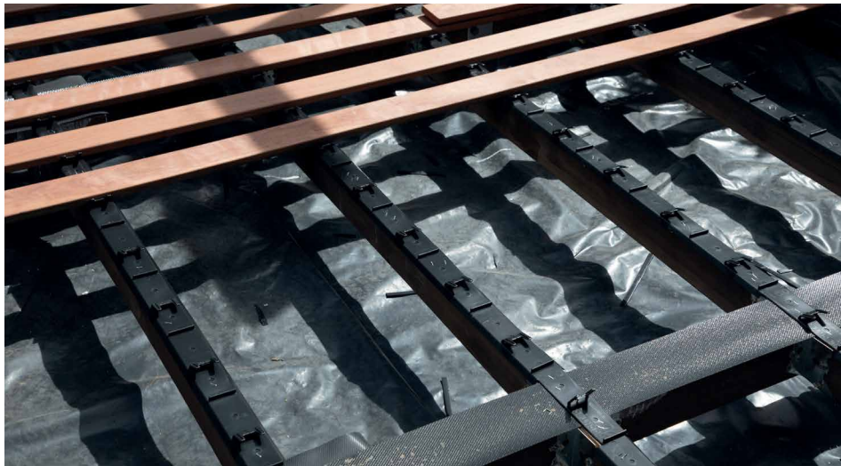
Above: Woodhouse have tested the product with a range of proprietary decking clip systems and found all worked well. Here a side-fastening system will deliver a smooth completed deck when finished.
