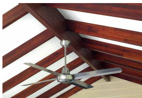
Above: Merbau timber used inside in structural applications is both strong and beautiful.
