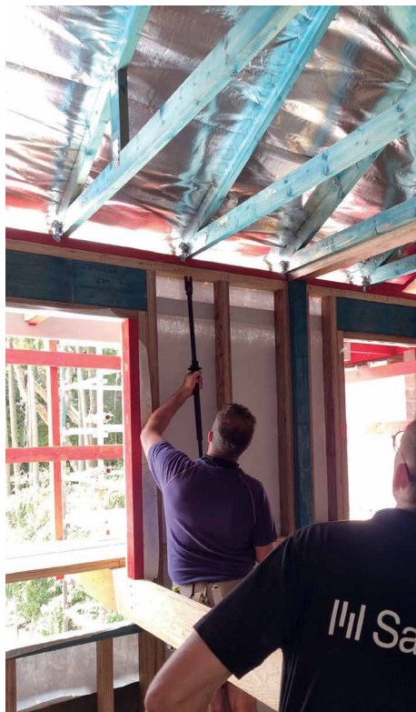
Above: Simpson Strong-Tie's Quik Stik system is easy to use in confined positions.
