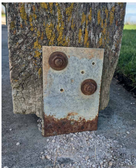
Above: Galvanised products aren't suitable for coastal sites like this picnic shelter as they rust and let rot into surrounding timbers. VUETRADE has often been called in to replace product like this with stainless steel.
