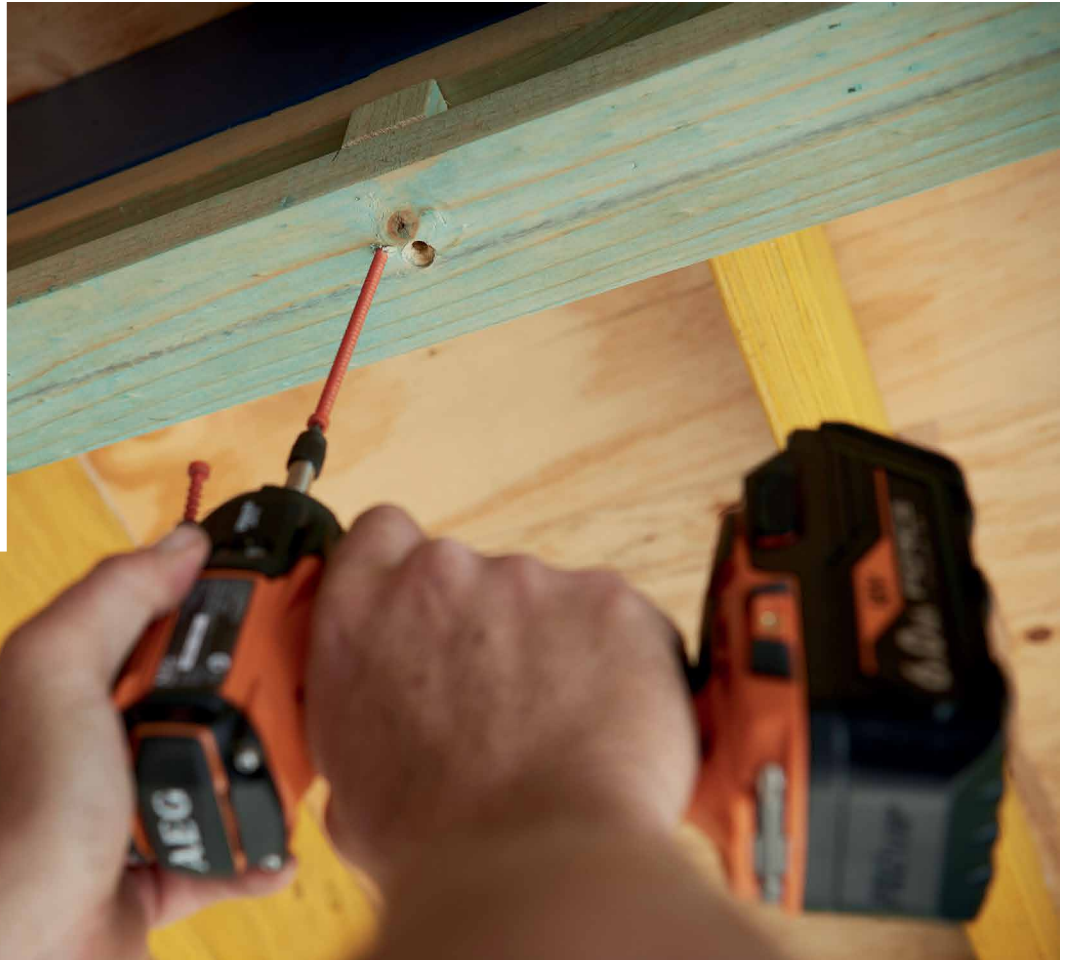
Above: Simpson Strong-Tie's SDWC truss screw replaces framing anchors for rafter and truss to top plate connections.
