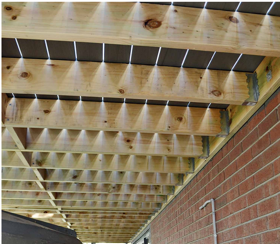
Above: Using the right joist hangers, like these from VUETRADE, will add years to your deck's service life.
