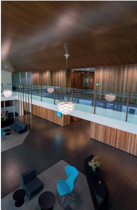
Above: Clear lacquered spotted gum lining board, installed by Wainwright Facades.
