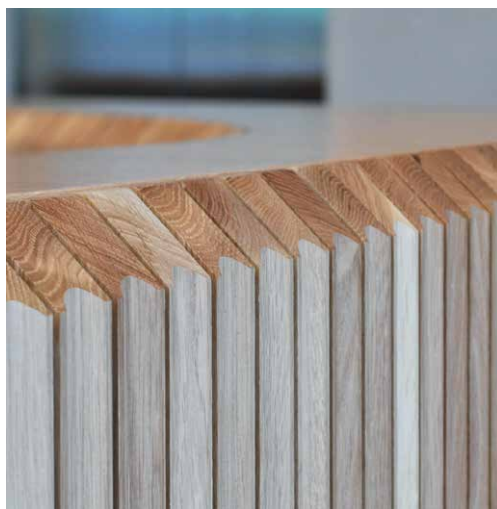
Above: Scallop-edges are popular; here in American oak custom screening by Timbeck for a new high-end office building, 100 Mount St, North Sydney.
