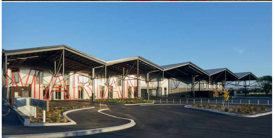
Above: Marian College: makes use of an existing warehouse by constructing a built-for-purpose timber school inside the original steel building. Architects: Sheppard & Rout.
