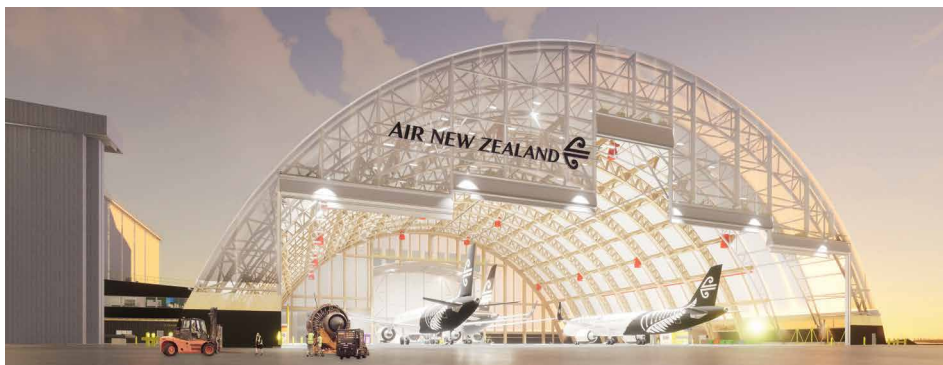
Above: Air New Zealand’s Hangar 4: at 98 metres, it will be the largest single-span timber arch aircraft hangar in the southern hemisphere.
