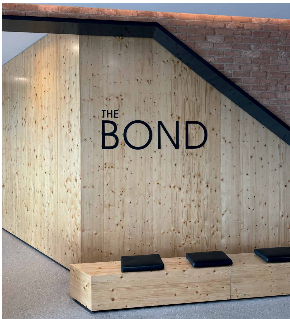
Above: The Bond foyer proudly displaying the building name on pine feature wall. Twelve months after opening, with the Intergrain UltraClear maintaining the original charters of the timber.
