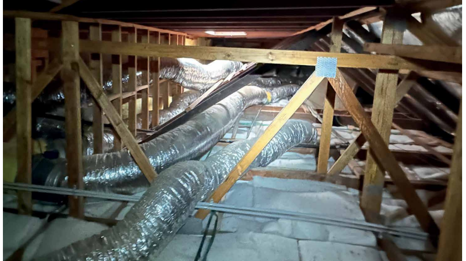
Above: The girder top chord was designed for 600mm restraints but it's more like 3m!
